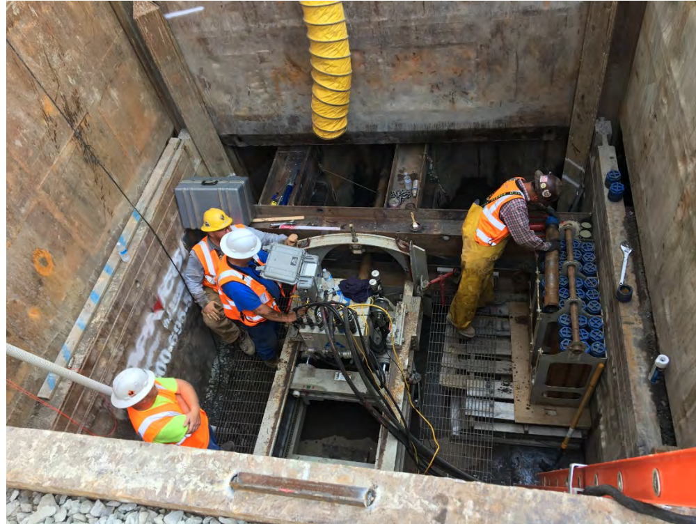
Pilot tube exploratory investigation
