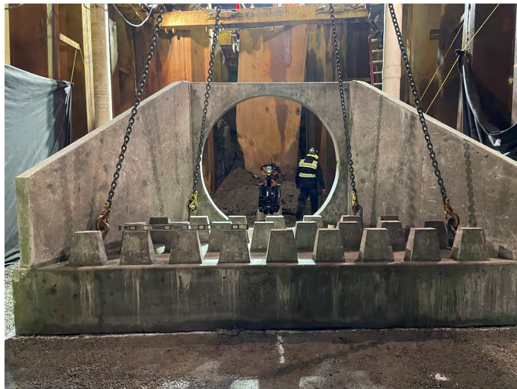
Outfall energy dissipater
